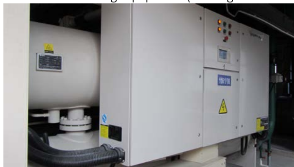
Advanced Air Conditioning Equipment (Cooling Water Machines)
